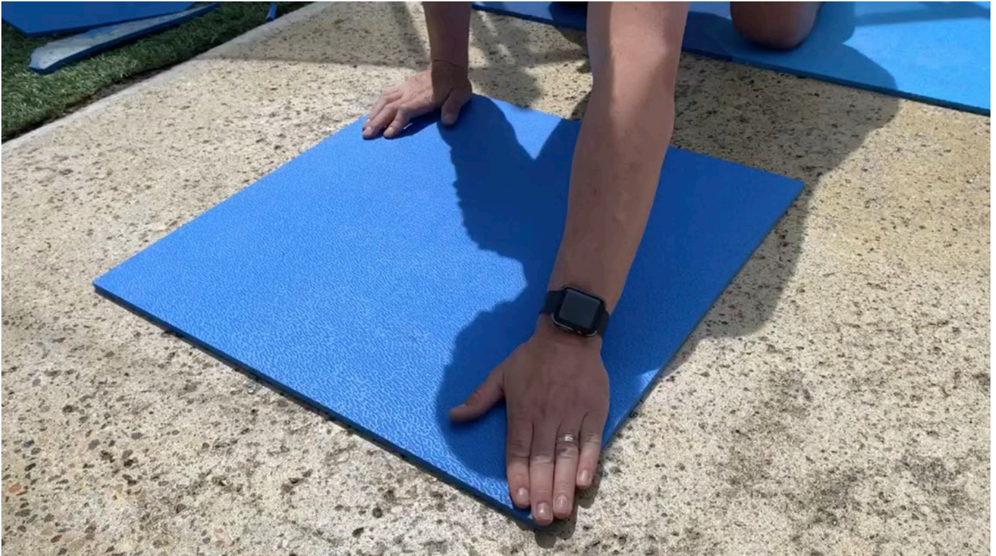
Step 3: Press down on the tile to make sure it's securely adhered to the concrete.
