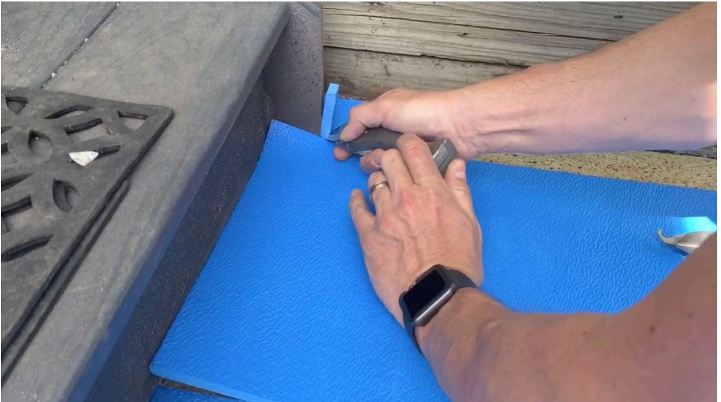
Step 12: Closely cut off the excess piece and press the tile down on either side.
