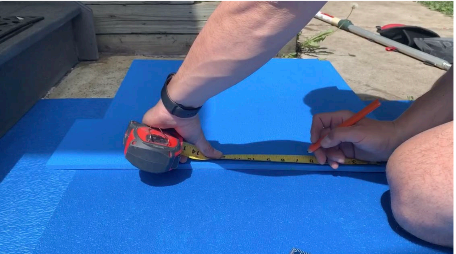
Step 7: Mark the two points on the tile and connect by drawing a line along a straight edge.
