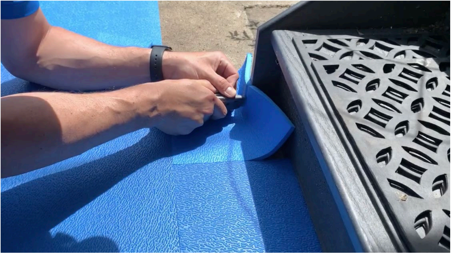
Step 15: Take a straight blade and run it along the vertical points.
