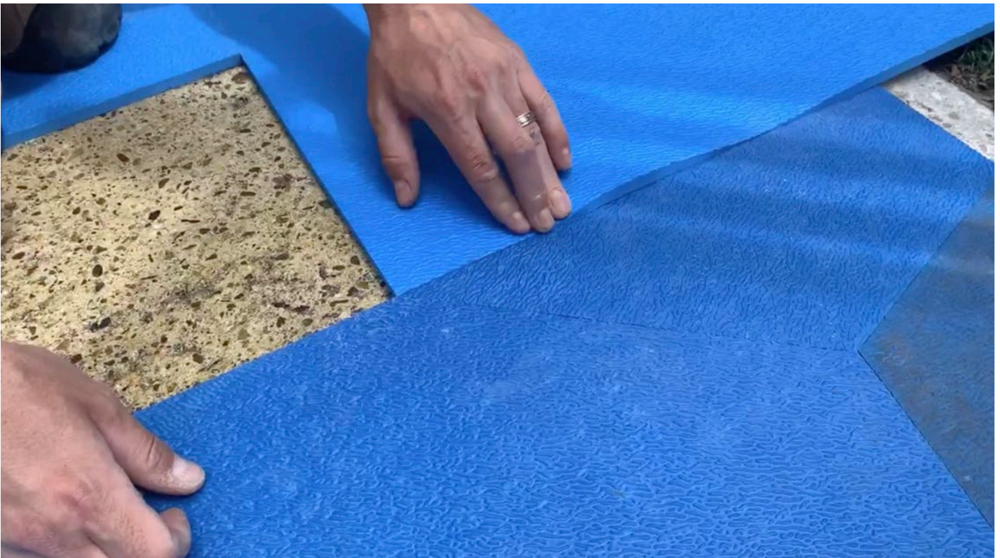
Step 8: Work the tile along the joints, ensuring a tight fit.
