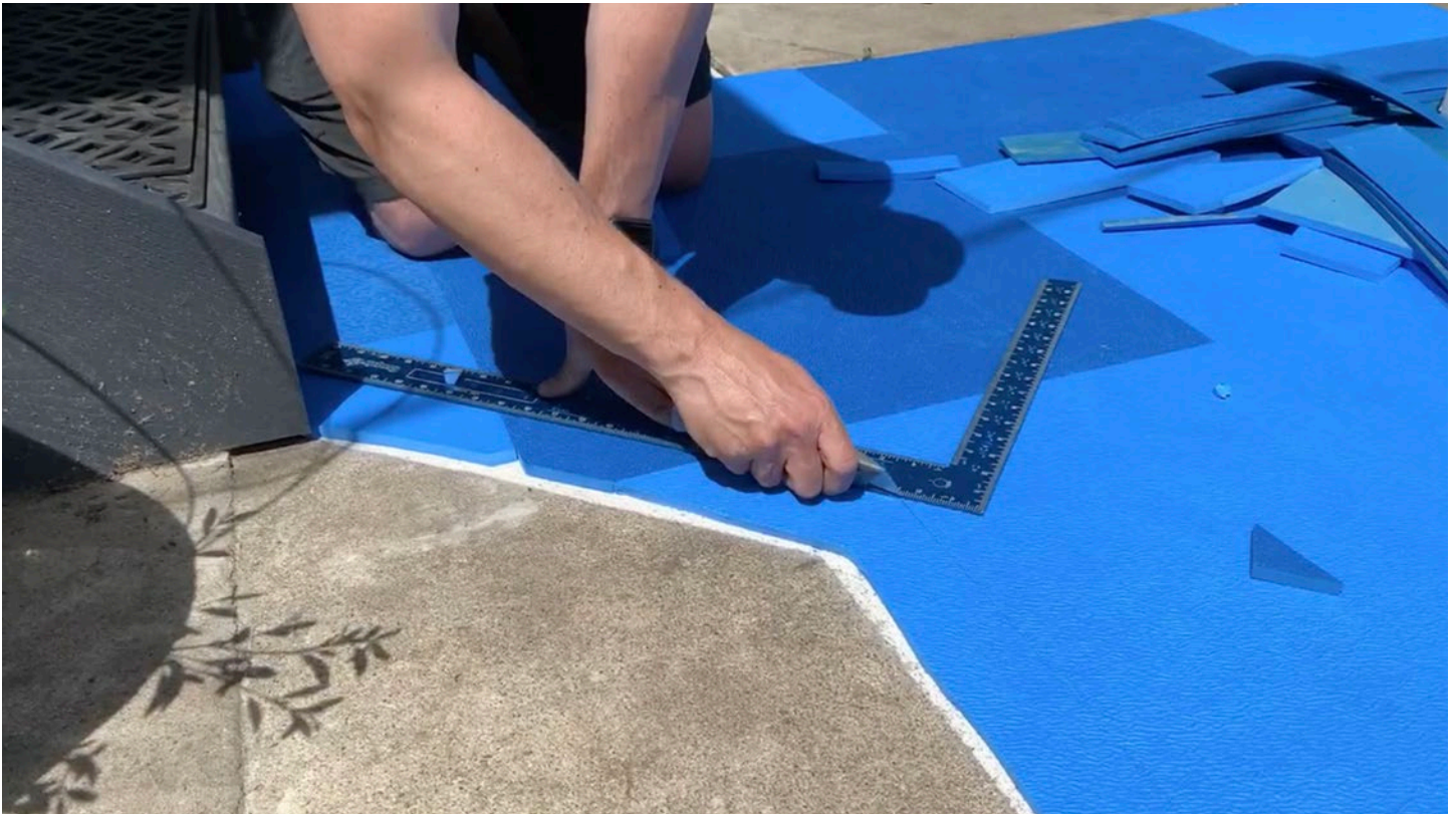
Step 21: Continue to cut along all lines from transition strip layout.
