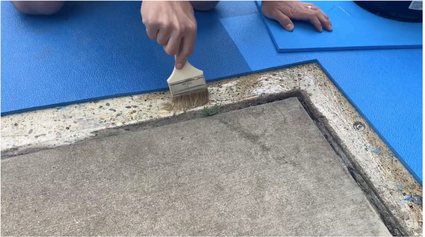
Step 25: Use a chip brush to get 100% adhesive coverage at the edges for Transition Strips. Keep the brush on the concrete, ensuring to not get adhesive on the sides or tops of the tiles.
