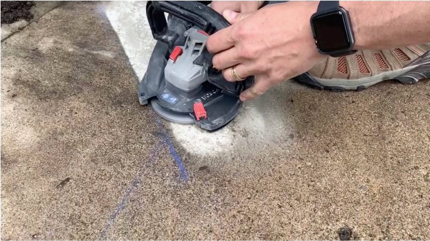
Pull back the guard on the grinder to get a crisp edge along the chalk line.
