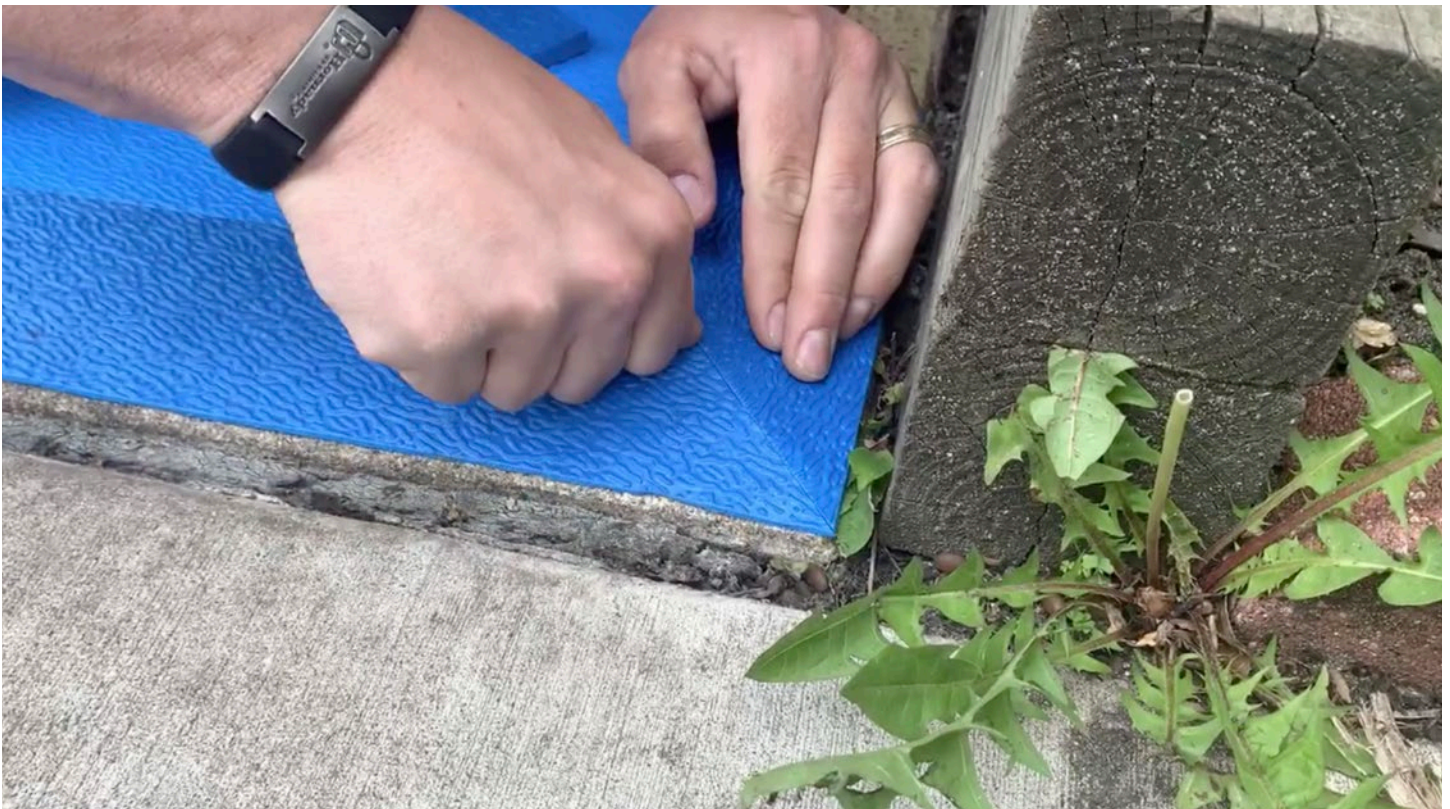
Step 32: Press down and ensure both joints line up tightly. Continue placing Transition Strips around project perimeter until it's fully finished.
