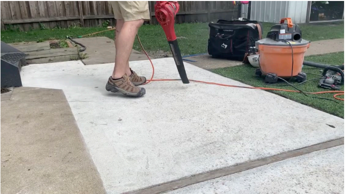
Step 3: Use a leaf blower to clear the surface of any dust or debris. Contaminants prevent the adhesive from properly bonding to the concrete and can lead to delamination after installation.
