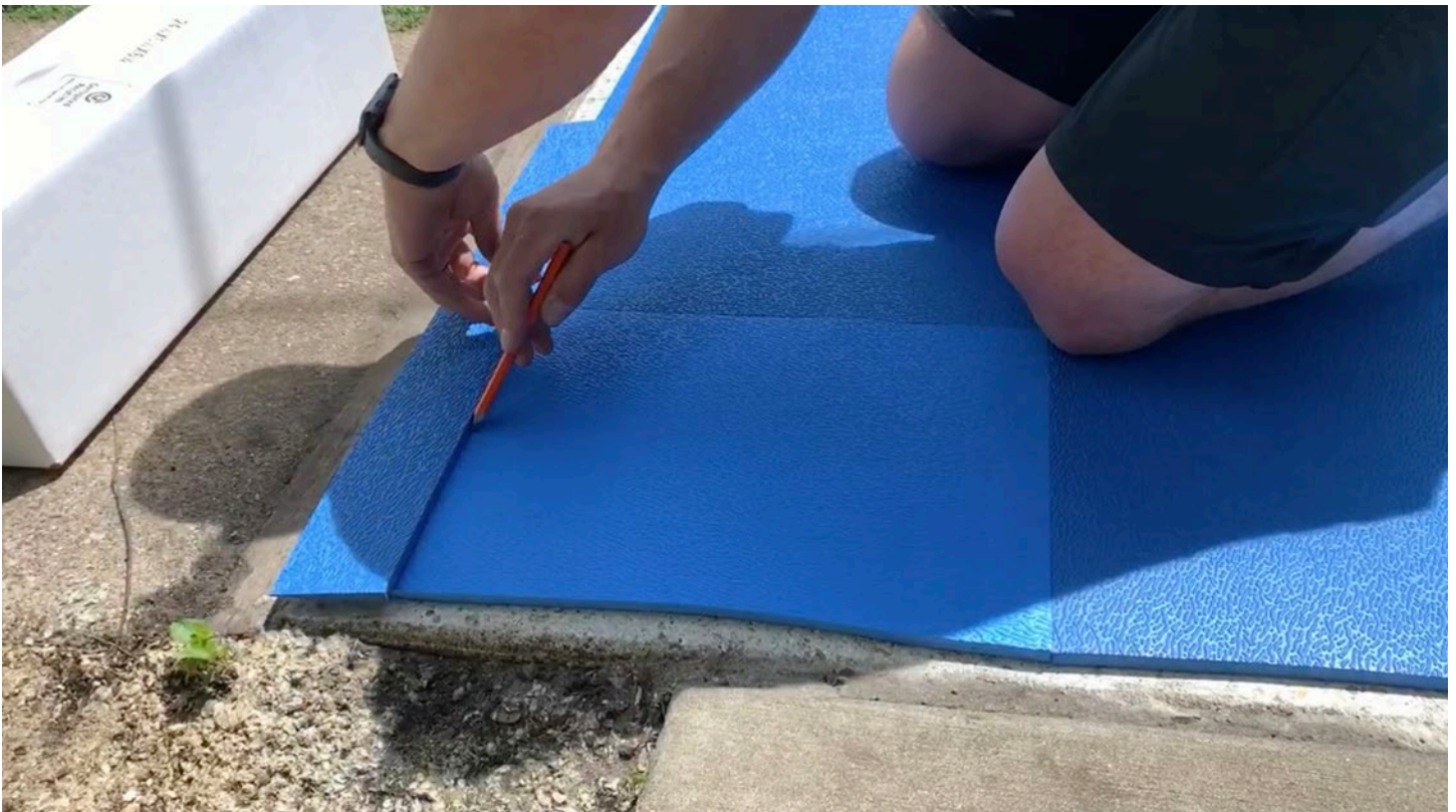
Step 19: Transition Strips will be mitered at the corners, so it's important to fully lay out and mark their placement in advance. Pre-measuring also helps to keep spacing accurate.
