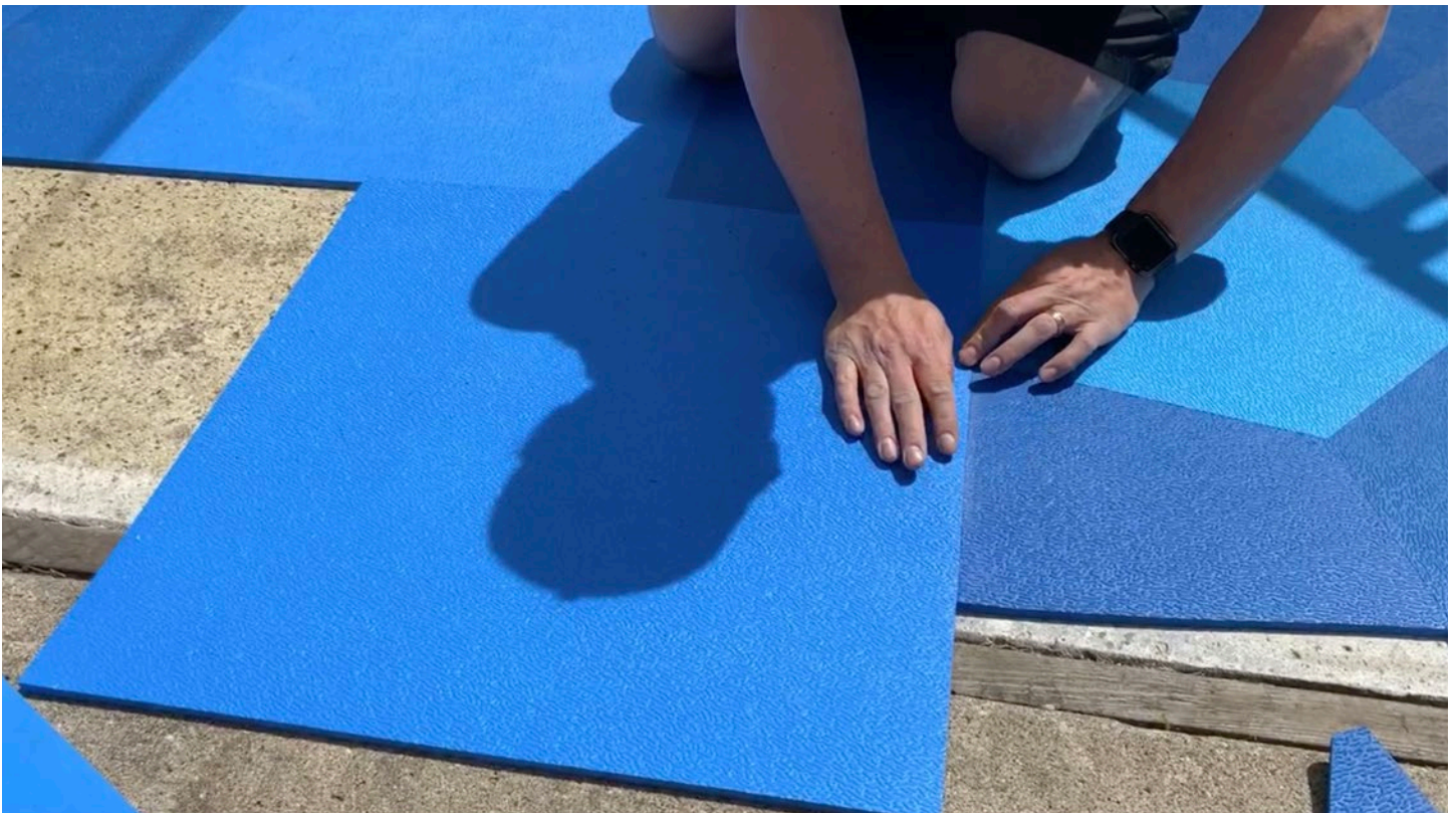
Step 12: Continue placing tiles to align with existing edges. After each tile is applied, press down across the entire surface to ensure a tight bond.
