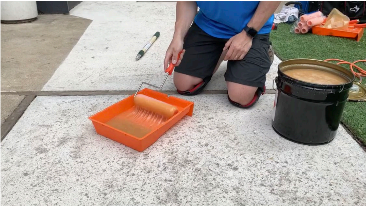
Step 3: Fill a sturdy paint tray and fully saturate a 3/8" nap roller.
