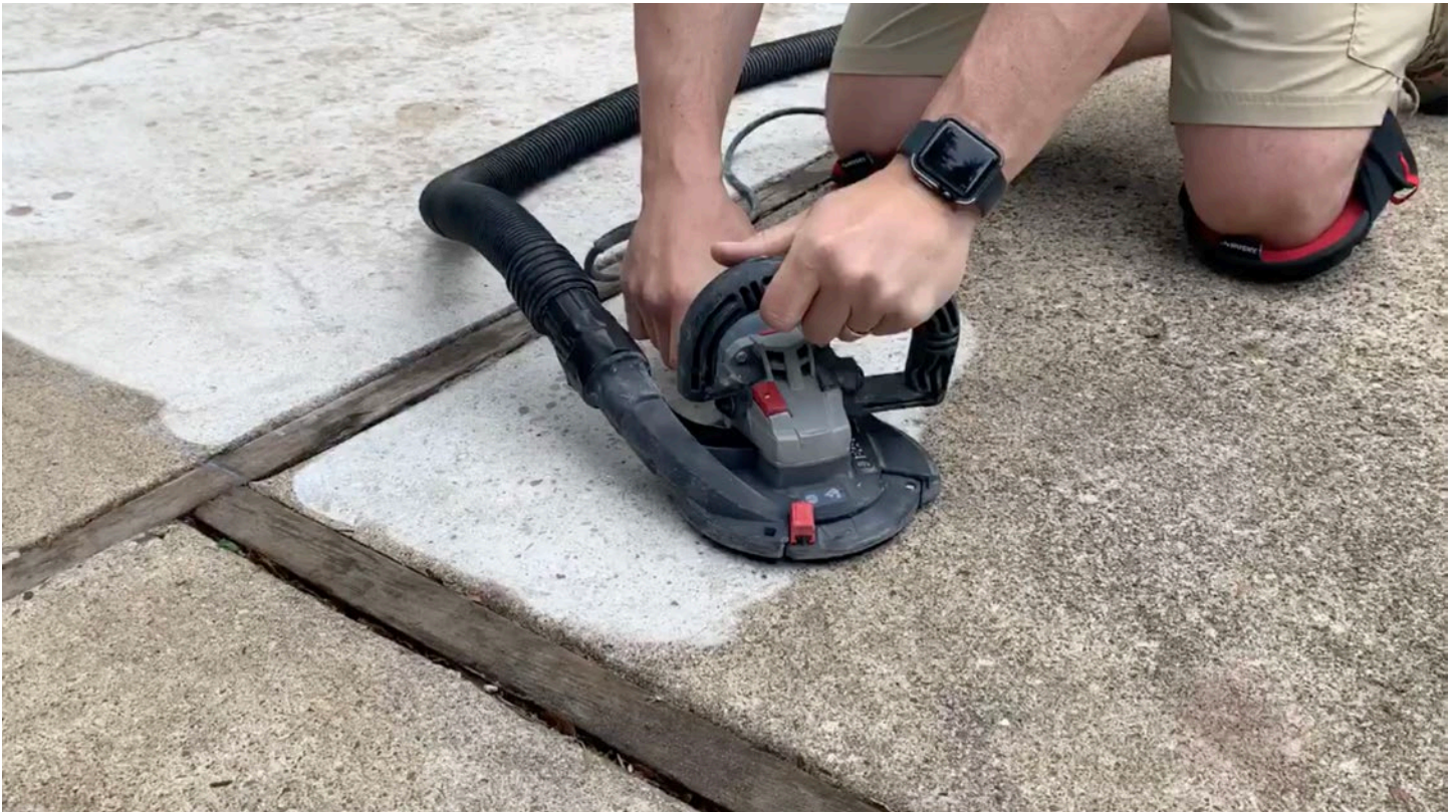
Tip: Attach grinder to a vacuum system to reduce ambient dust in the space and minimize clean-up required at the end of the preparation stage.
