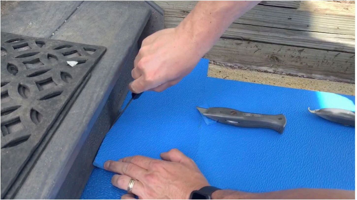
Step 13: Tuck tile below the step using a putty knife for a clean finish.
