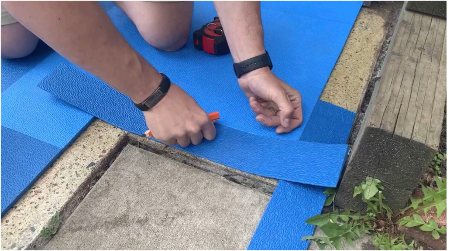
Step 29: Place the perpendicular piece to lay over the first transition strip at the corner for mitering.
