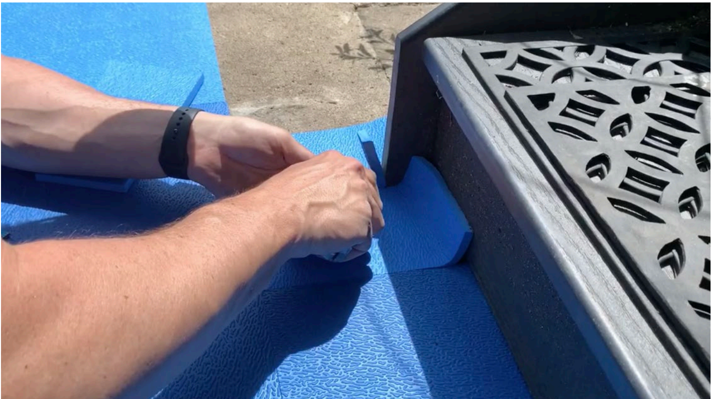
Step 16: Push the tile down and trim off any excess.
