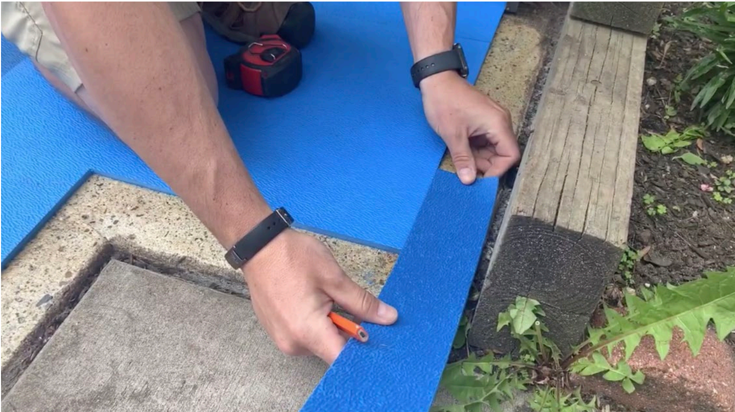
Step 28: Place the transition strip down, butting it up tight against the edge of the tile.
