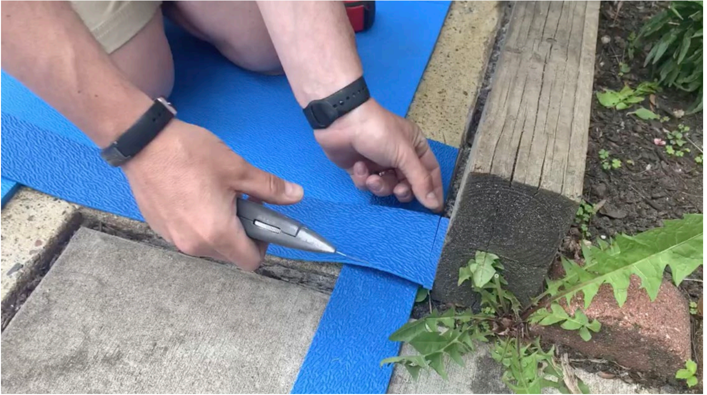
Step 30: Cut off any excess as needed, leaving enough length for the miter.
