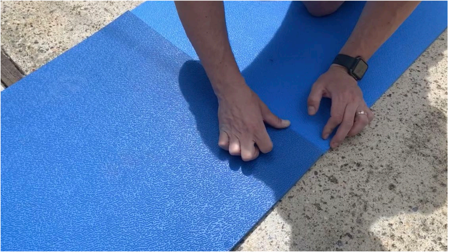
Step 5: Use your thumb to work the tile into the joint in order to ensure a tight fit.
