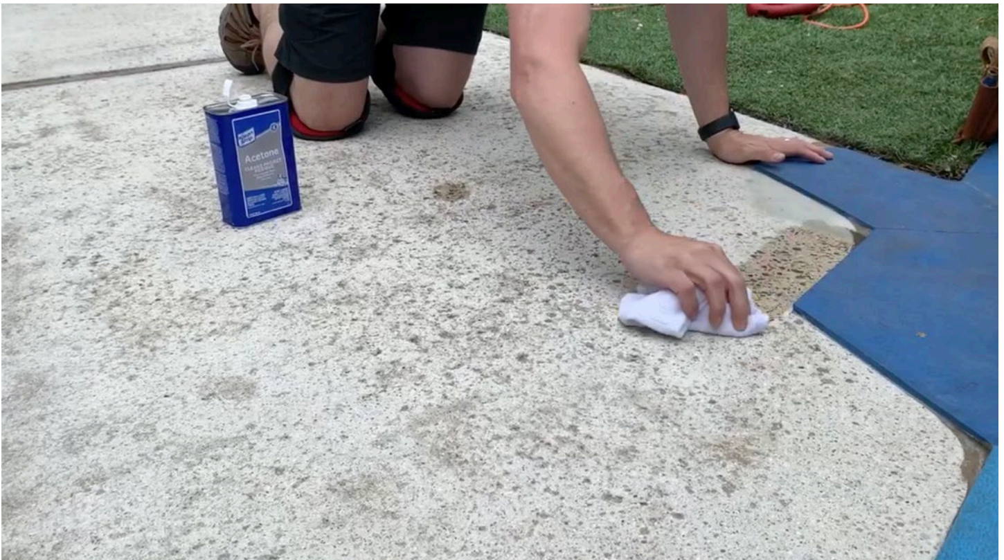
Step 4: Use acetone on a rag to thoroughly disinfect the surface. Acetone permeates the concrete pores to remove any remaining debris or fine particulates.
