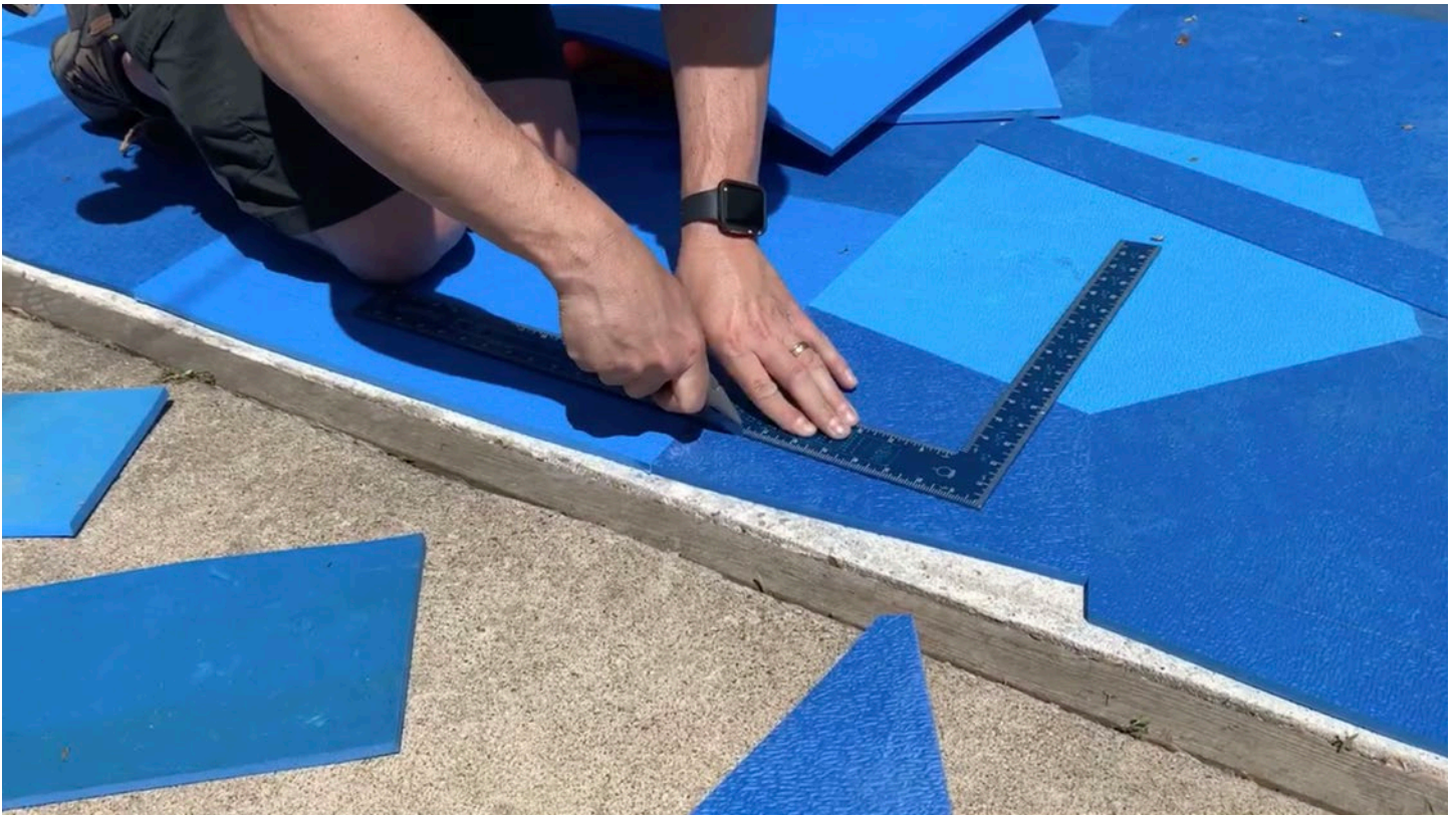
Step 20: Once measured, cut lines along a straight edge. If you're right-handed, cut with excess to your right to create a natural bevel with the blade. Do the opposite if left-handed.
