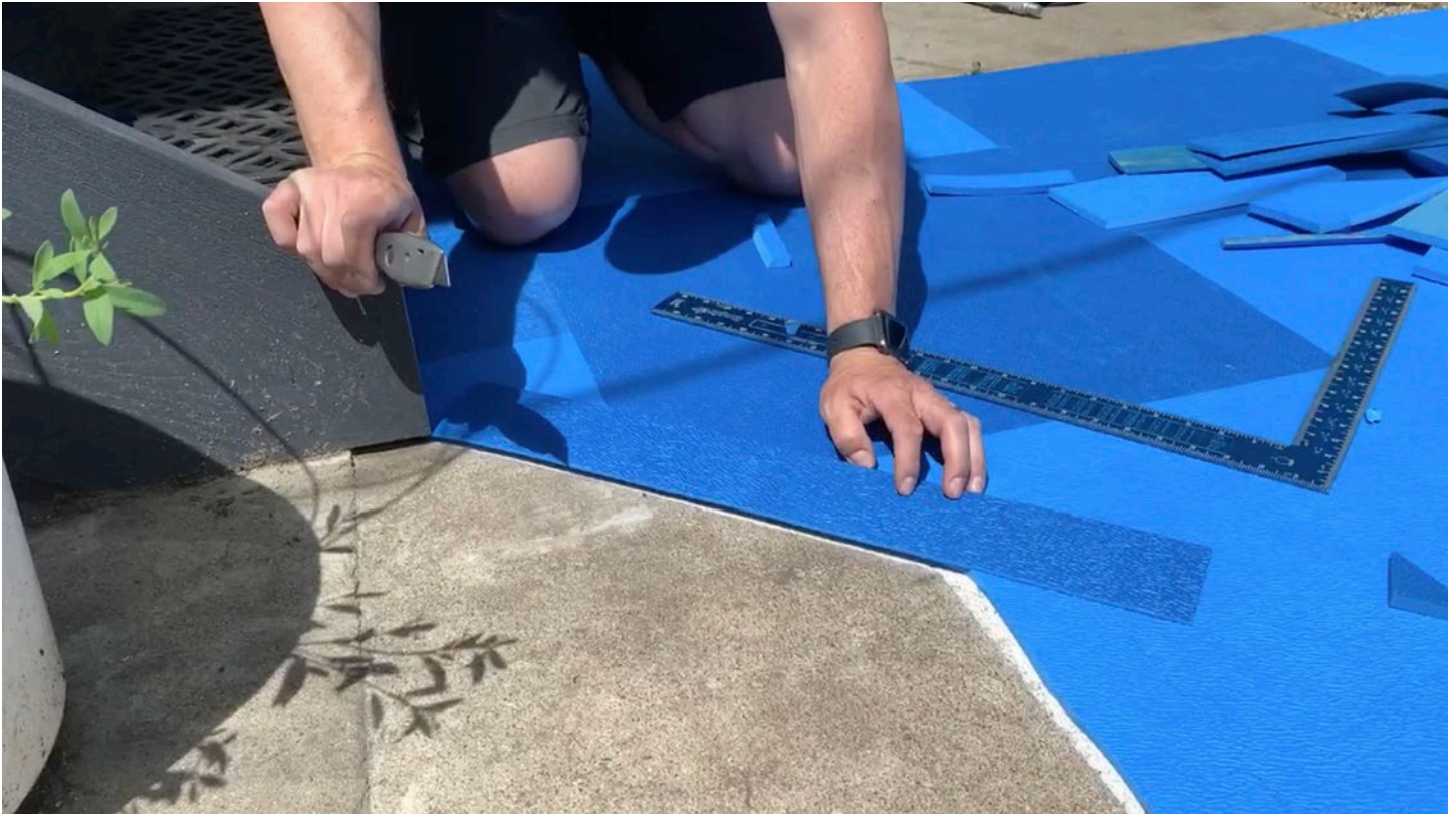
Verify the distance is accurate where Transition Strips will end.
