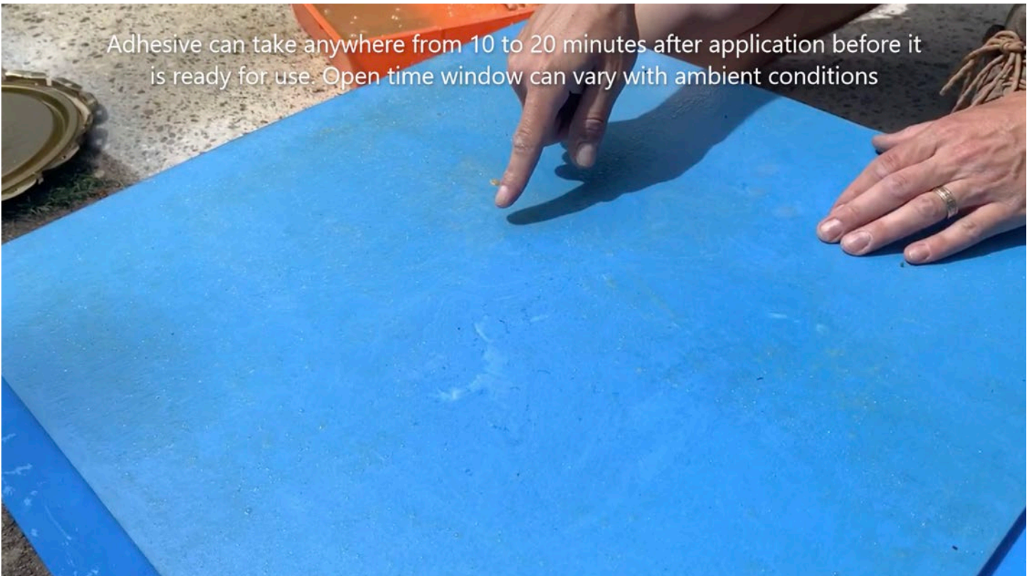
10-20 minutes later, check to see if adhesive has cured. If it's gooey and transfers to your finger, it's still too wet. It's ready once it's tacky and doesn't transfer to your finger.
