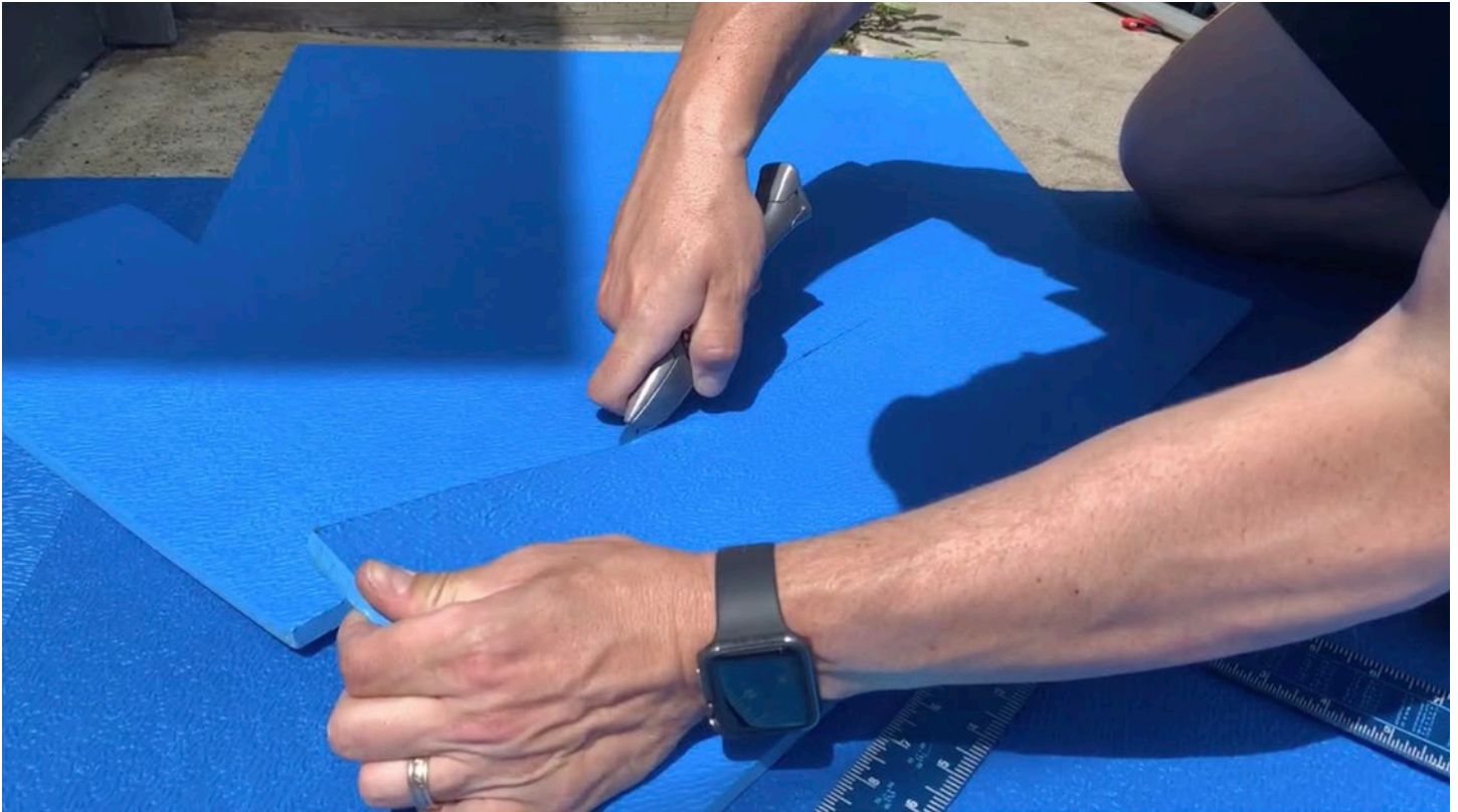
Step 9: Cut with a large hook blade, keeping the tile lifted slightly. This prevents anything below from getting damaged. Ideally, use a cutting board if you have access to one.
