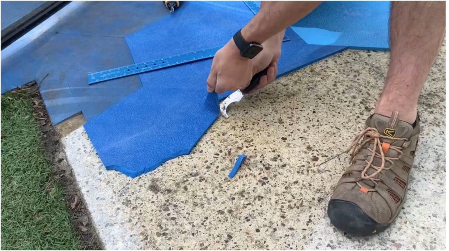
Step 8: If needed, peel up any tiles previously glued down on the other side of the cut line and use a stiff putty knife (or a 5-in-1 tool) to get underneath the tiles for removal.
