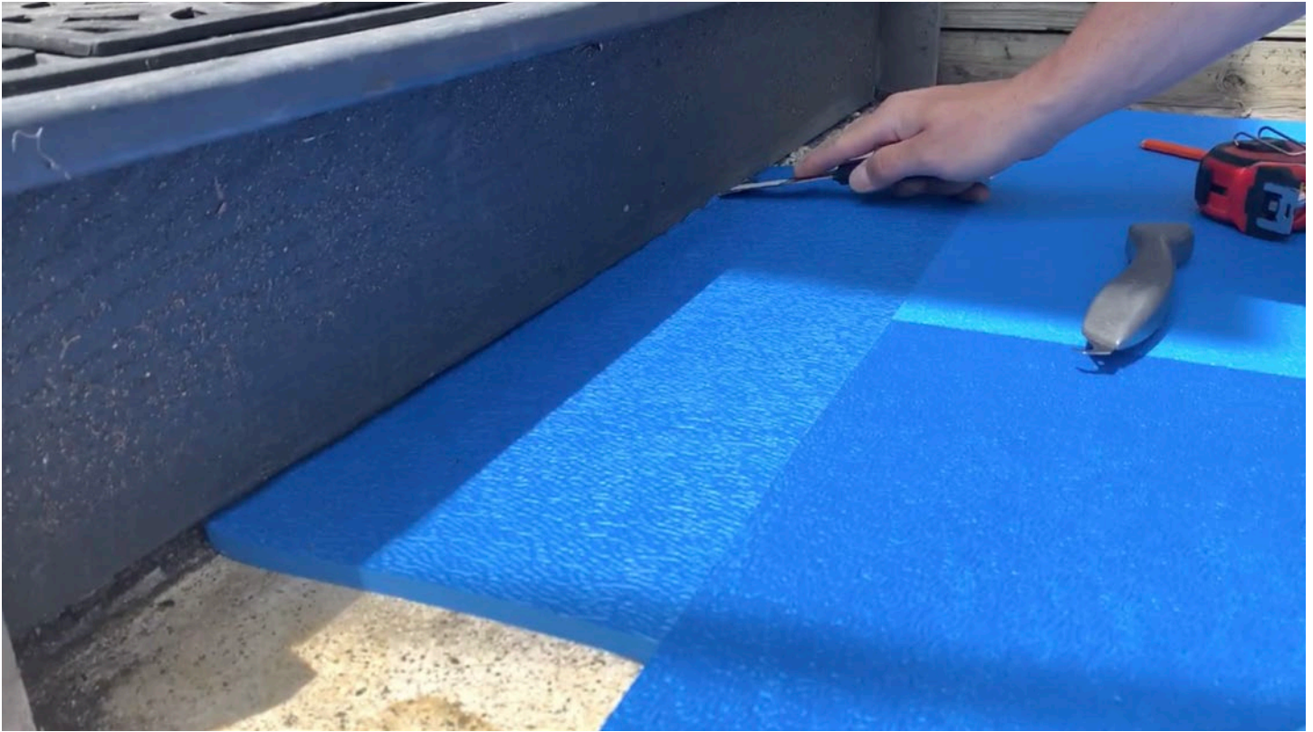
Step 5: Tuck the tile below the stair riser and use a 5-in-1 knife tool to work the pinch points down.
