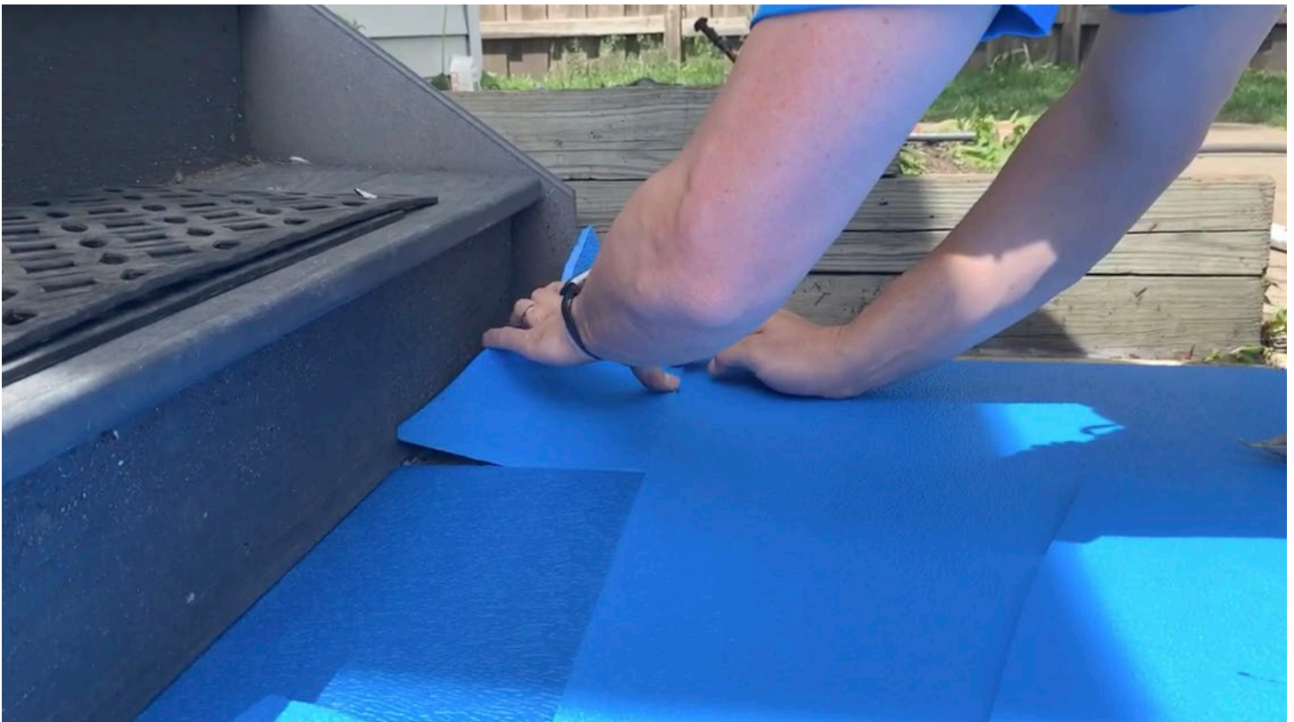
Step 10: Place the tile piece, keeping joints tight on the inside.
